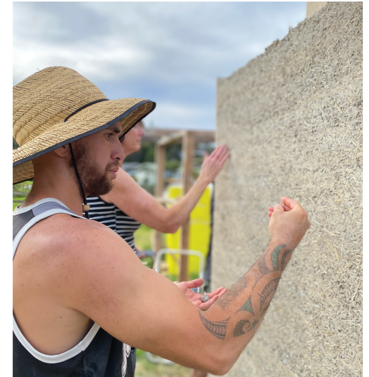
A new pātaka kai was built using hempcrete at the Marfell Community Garden as a demonstration build, while gifting a taonga to the community.
